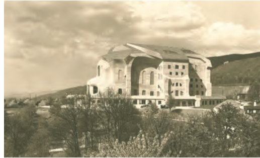
The second "Goetheanum": flowing reinforced concrete.
